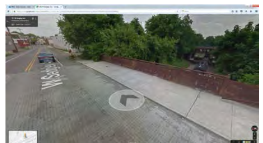
Overpass at Sedgley and Freight Rail
