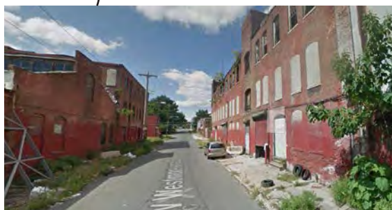
Vacant industrial plants and street. The public realm shows maintenance as poor as the buildings. Broken sidewalks, overgrowth, few street lights, no wayfinding or street signage.
