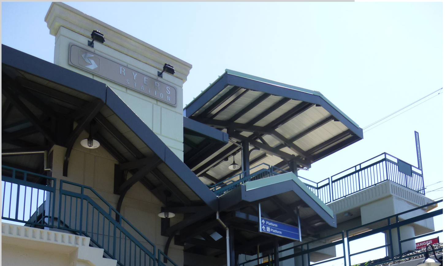
Ryers Train Station
